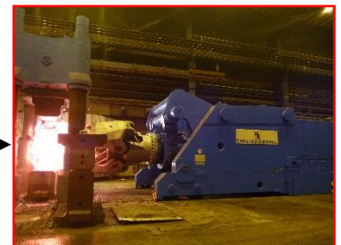
Many 80 ton machines have been installed by DDS during past decade.
